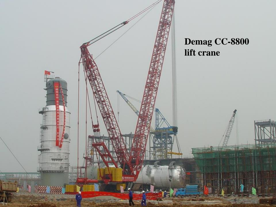
Note the hydraulic stinger for changing the radius of the superlift from 19m to 25m
